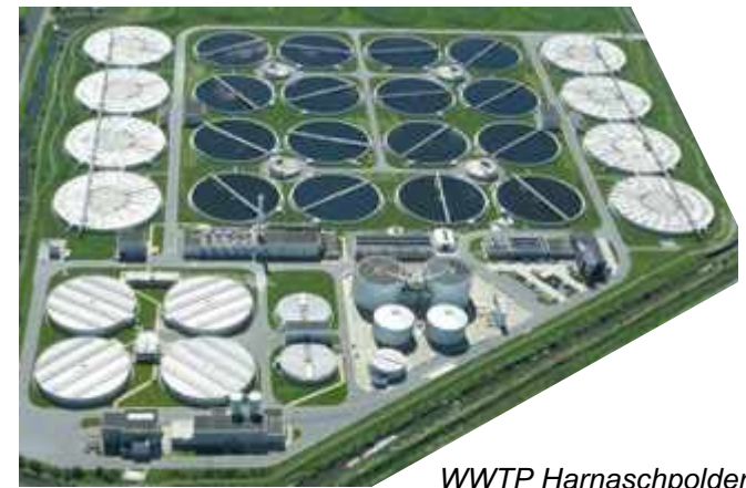
WWTP Harnaspolder - Delft
